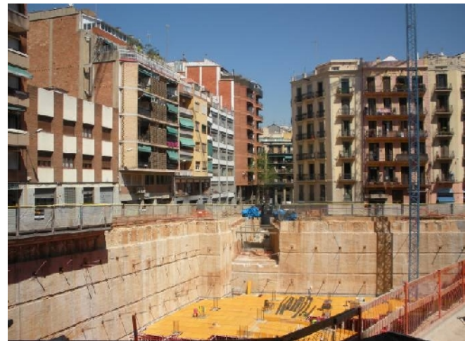
Photo 30: Construction of an underground car park and remodelling of Plaça de les Navas. (A.M.)
