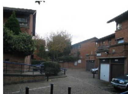
D'Eynsford Estate, 1960s housing estate located north of the Lettsom Estate
