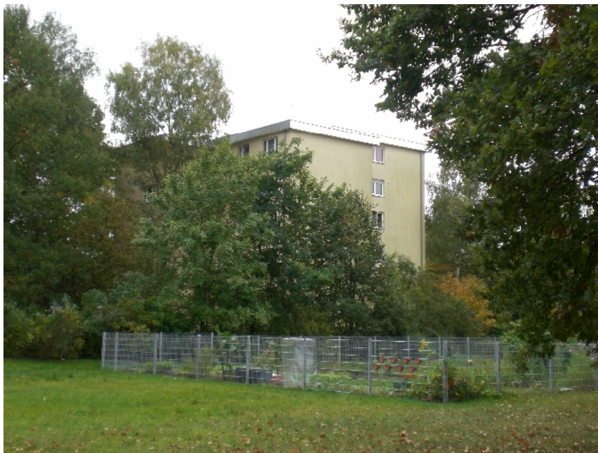
Pic. 2.1 Part of the Intercultural Garden Langwasser with housing development in the back
