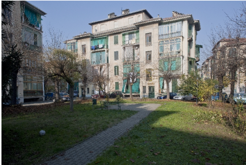
Fig. 3.2 Internal view of social housing complex
