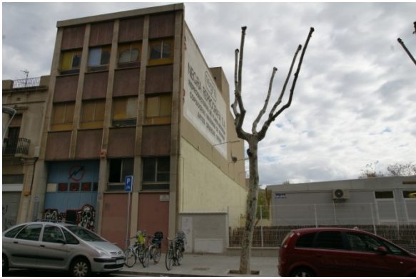
Squatted property located next to a primary school (Castillejos Street).
