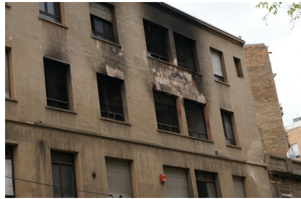
Another squatted property / supposed illegal warehouse that was recently set fire (Consell de Cent Street).
